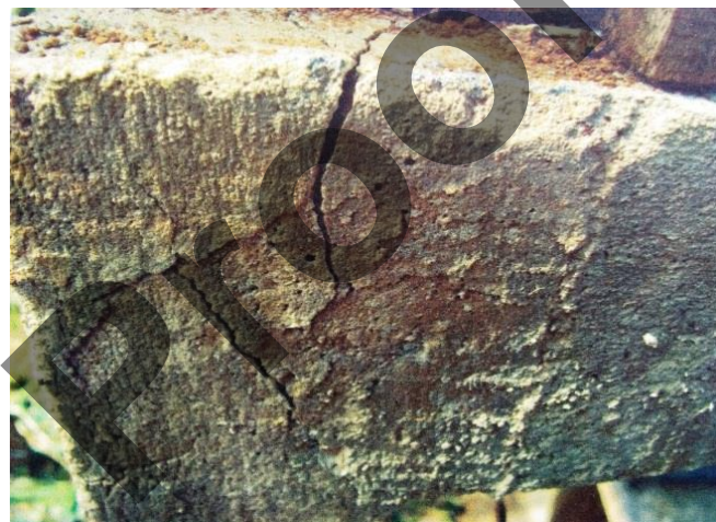
Fig 6: Cracks noticed on the beam/column joint
