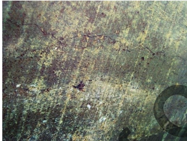
Fig. 5: Yield line pattern noticed on slab
