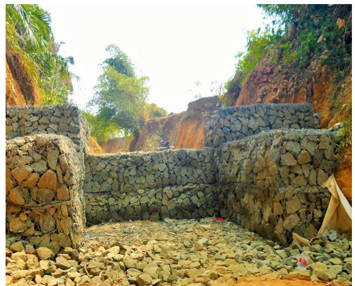
Figure ( 5 ) Gabions and Reno Mattresses used to protect infrastructure in vulnerable site
