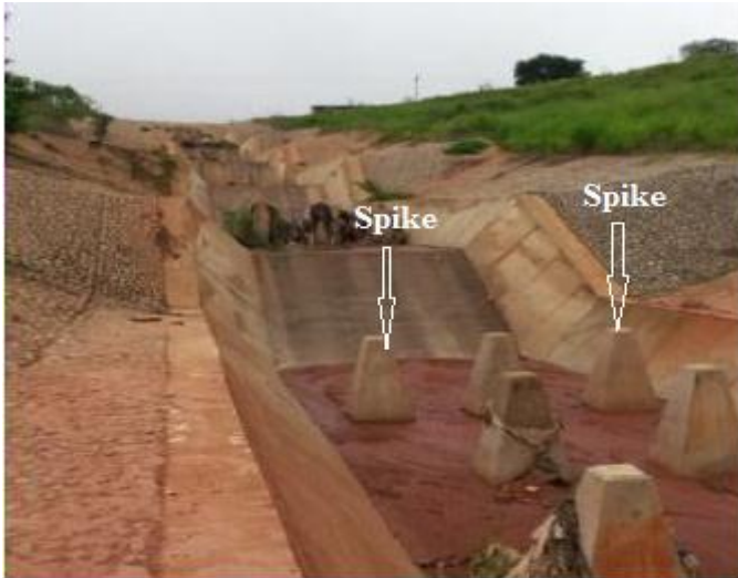
Figure ( 3 ) Step wise drop, chutes and spikes
