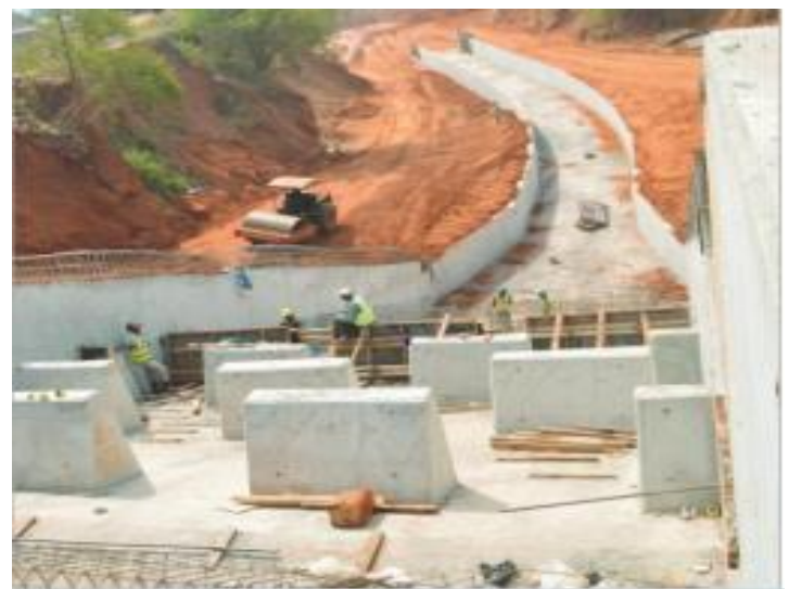
Figure ( 6 ) Spikes preventing undue acceleration of flow and dissipating energy.
