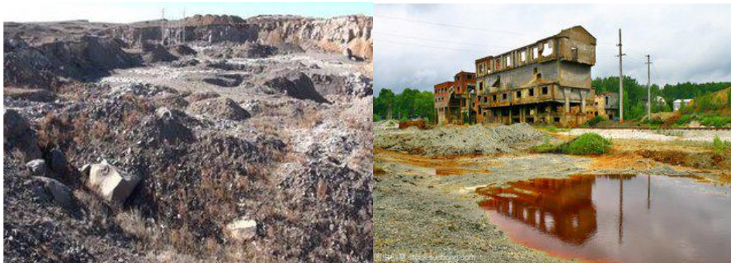
FIG. 1 An Abandoned Mine In A Certain Place
