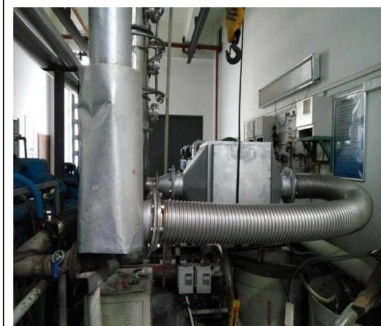
Fig 4. exhaust coolers.
